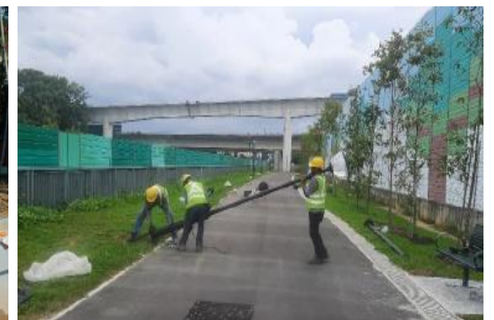
Installation of lamppost for PCN
