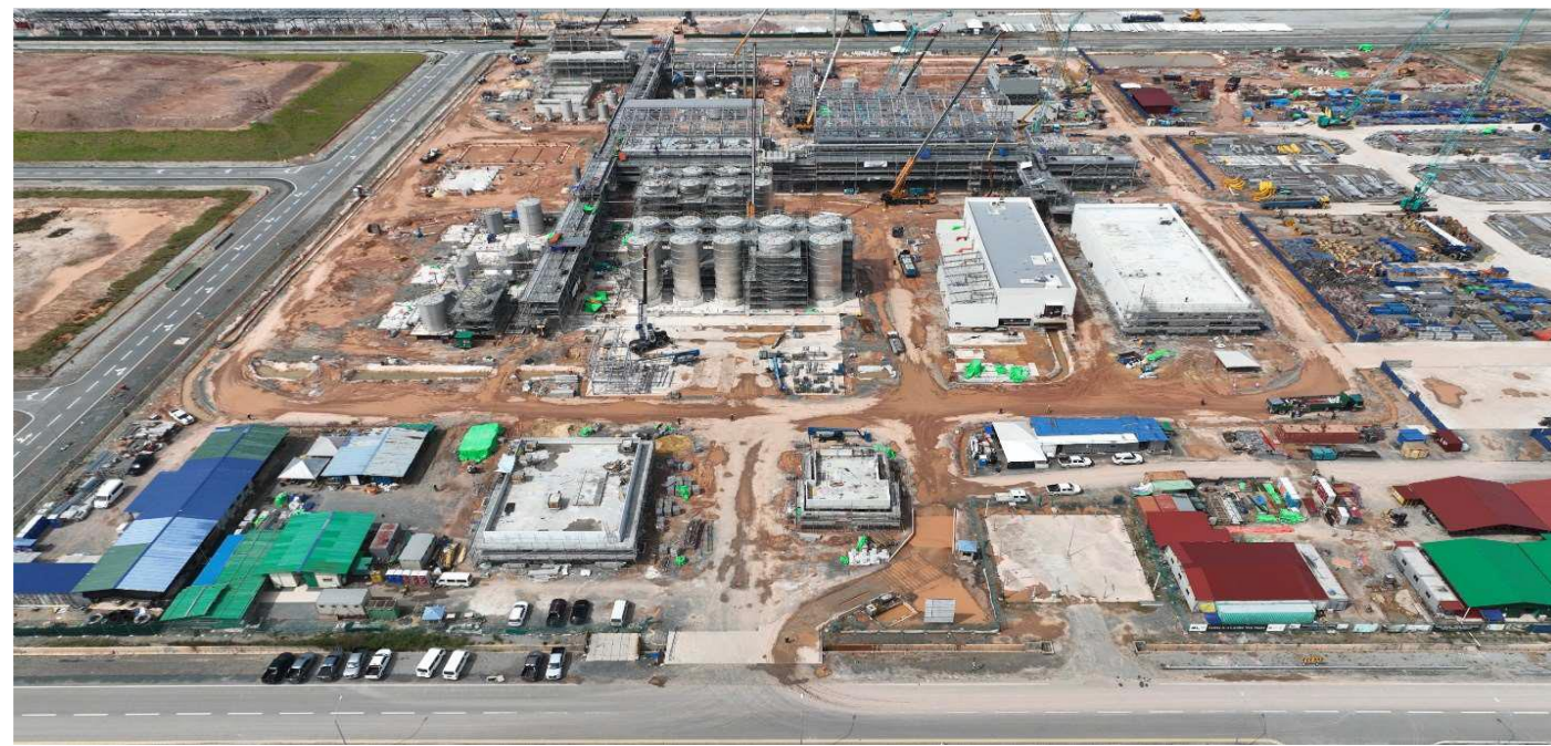
Overall NBL project site
