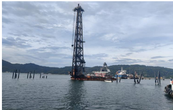
Positioning for SGP 3 for piling work
