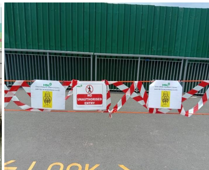
Signages to warn public of works ongoing at the PCN
