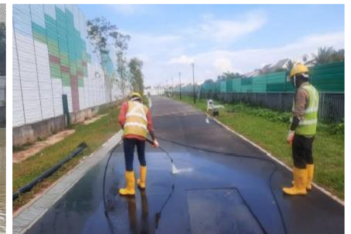
Cleaning of PCN Surface before handing over
