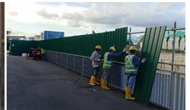
Installation of hoarding to successfully handover part of PCN
