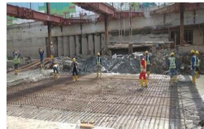
Construction of new Base Slab
