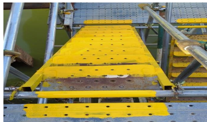
Slip trip hazards identified by painting yellow at common Access Egress
