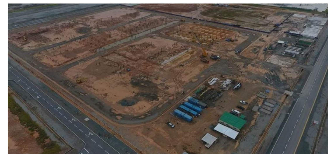
Overall NBL project site photo inside the PIC
