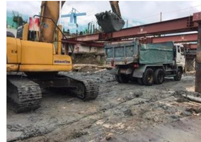
Clearing of soil within the canal
