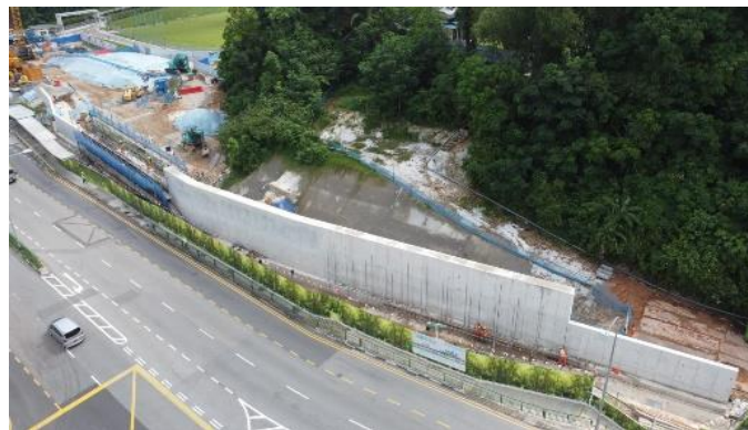
Retaining Wall Construction
