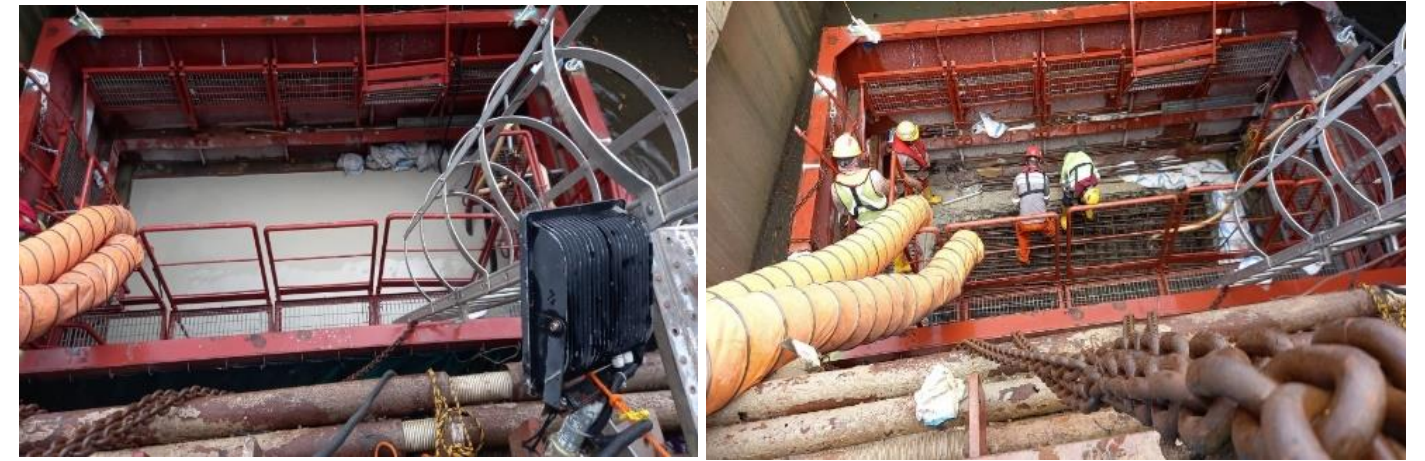
Base Slab Reinstatement works
