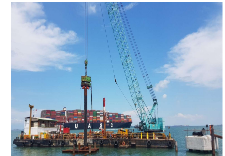
Staging Piling Method
