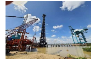
SGP 3 Pile Driving
