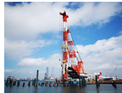
Piling Barge Method
