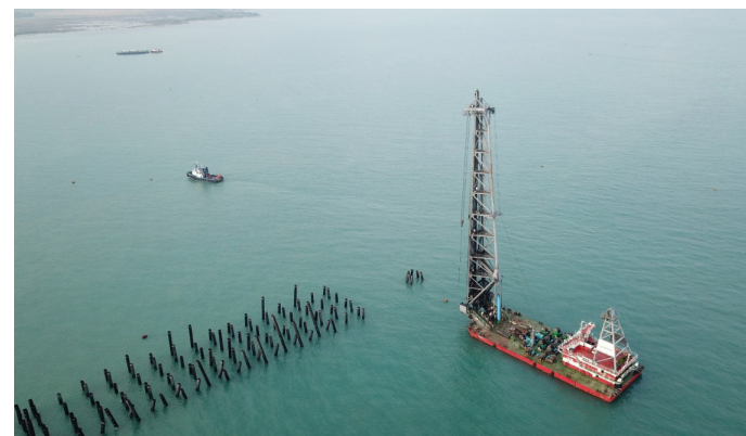
SGP3 driving the last pile of TJB56
