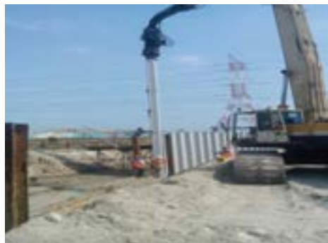
Vinyl Pile Driving
