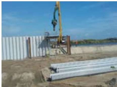
Vinyl Pile Driving
