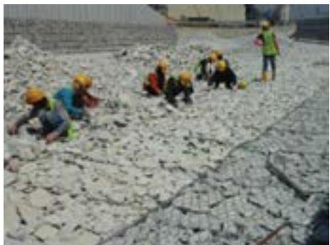
Mattress Preparation in Channel
