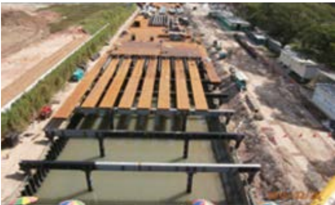
Installation of metal decking
