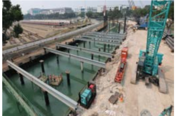
Piling stage of project
