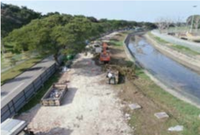
Initial stage of project
