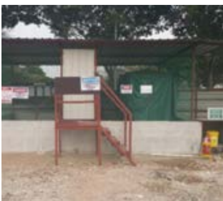
Chemical storage area with bund wall and SDS clearly displayed for end user to be aware of hazards from chemicals.
