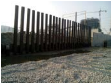
Permanent Steel Sheet Pile Driving
