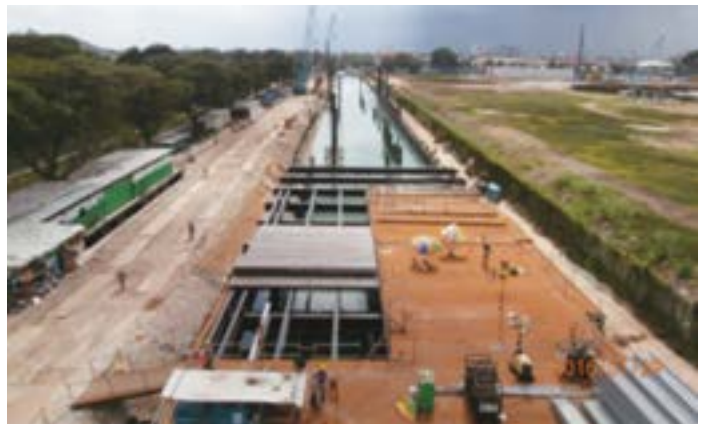
Installation of metal decking
