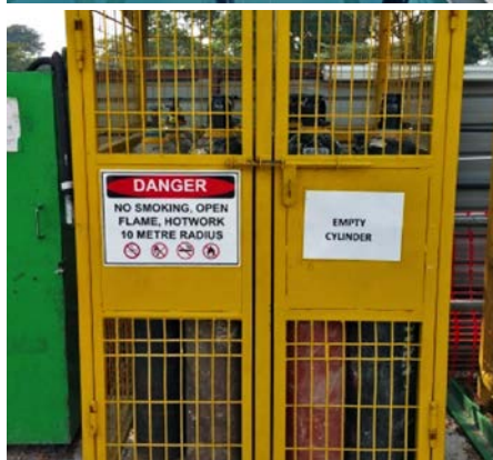
Good Housekeeping on Site – Proper cylinder storage area with locks and chain for securing
